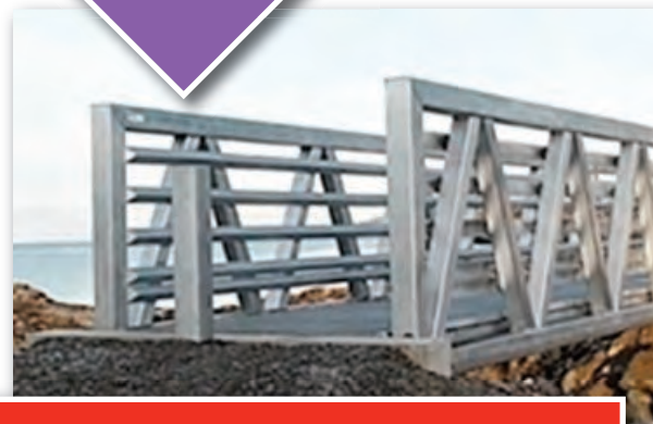
The Quaqtaq bridge in northern Quebec, Canada is a pony-truss bridge made of 6061-T6 aluminum extrusions. Courtesy of MAADI Group Inc.
